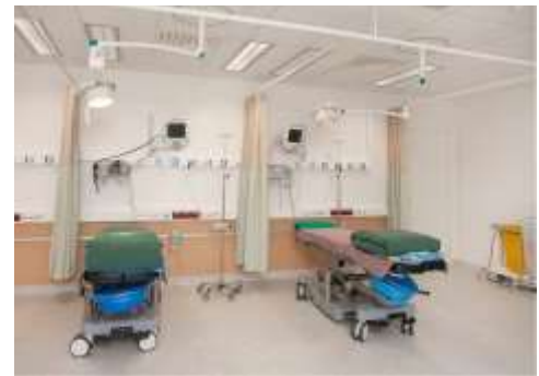
Lefkoşa State Hospital Recovery Suite refurbished
