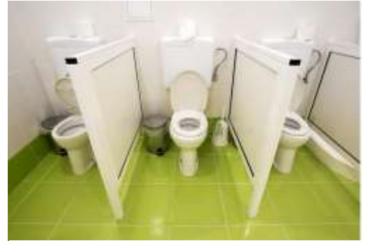
Lapta Primary School toilets refurbished
